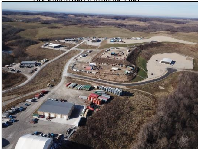
East Ohio Regional Industrial Park in Belmont County serving oil/gas industry. Photo by: Belmont Co. Port Authority
